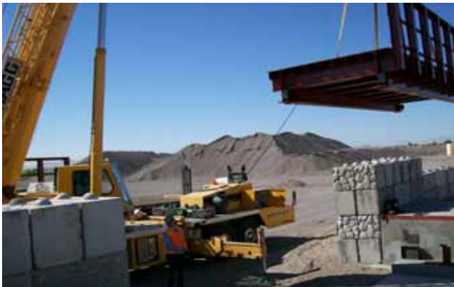
Figure 1 is placing the truck scale module in place
