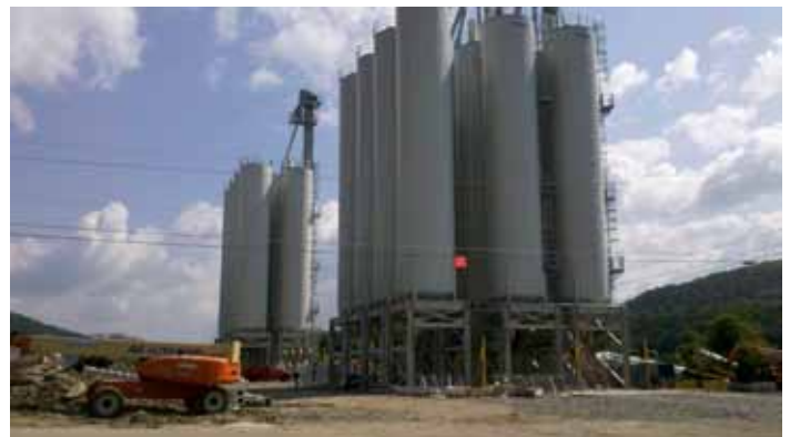
View of all silos containing fracking sand, to load and distribute to various drilling sites
