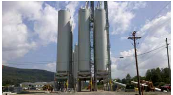
Fracking sand silos
