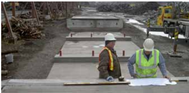
Figure 4 of preparing for scale installation
