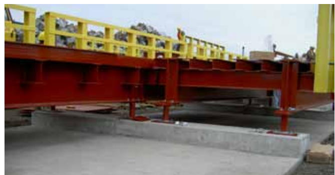
Figure 7 of new scale installed
