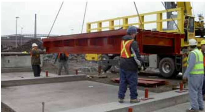
Figure 5 of new scale ready to install
