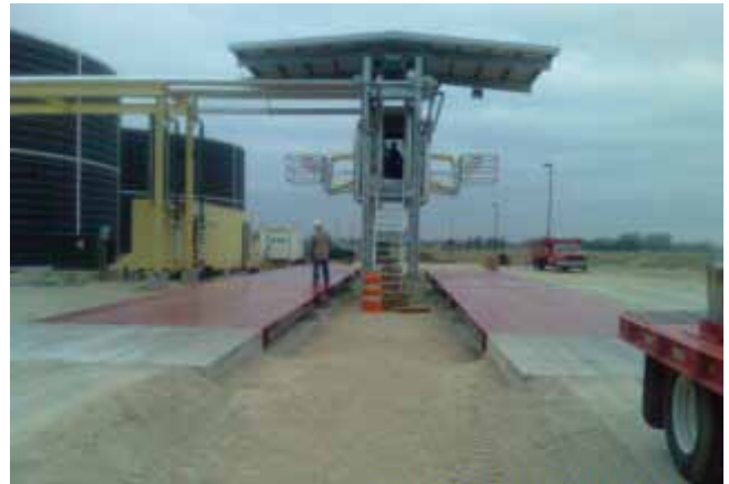
Figure1 of the MGQ facility
