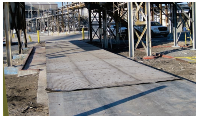
Figure 7 of new scale installed
