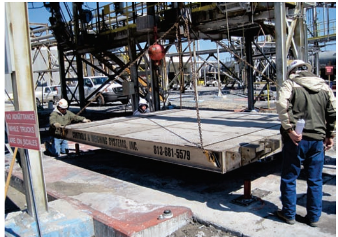
Figure 6 of new scale installation
